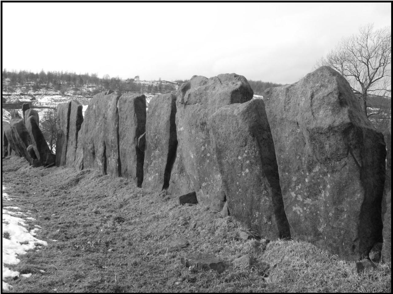
'A row of giant jagged teeth against the sky'. A section of vaccary walling on the fell side above Wycoller Dene. February 2010.
