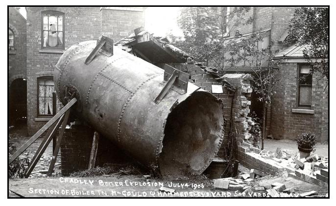
The five ton section of the Egg-Ended boiler that landed in Messrs. Gould and Hammersley's Yard. The roughly improvised section and plate brackets riveted onto the boiler shell are the mounting brackets that would have sat on the brick walls of the flues.
