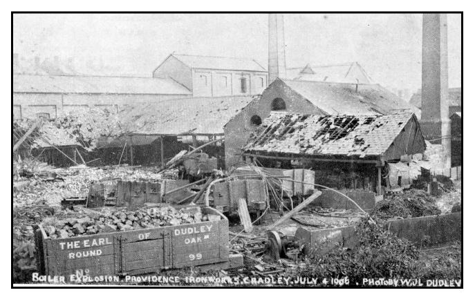
This interesting photograph clearly depicts the massive amount of damage caused to the roofs of the Ironwork's structures and buildings, with masses of roofslates having been ripped off, and significant volumes of brick debris scattered amongst the railway waggons in the yard.
