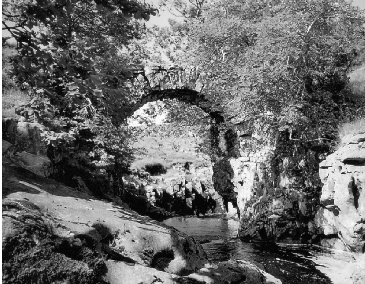
The crudely-built limestone semi-circular arch of Thorns Gill Packhorse Bridge which spans the deep chasm in the limestone that the Gayle Beck rushes down on its way to join the River Ribble. July 2004.
